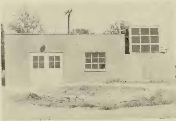
FILTER PLANT—MUNICIPAL WATER PLANT
